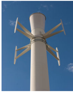
Ericsson Tower Tube with Wind Turbine Source: Ericsson
