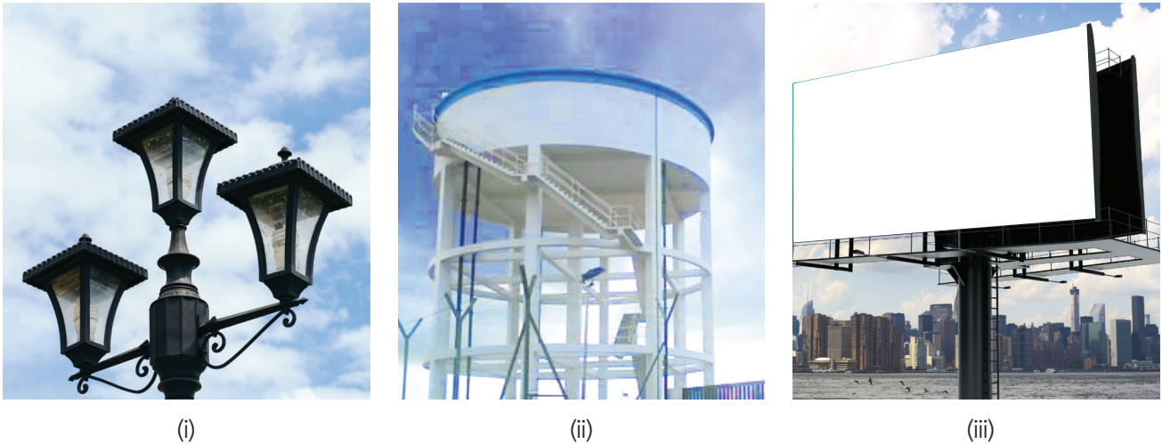
Figure 3: Example of Dual Function RCI (i) street light pole; (ii) water tank; (iii) advertising board.
