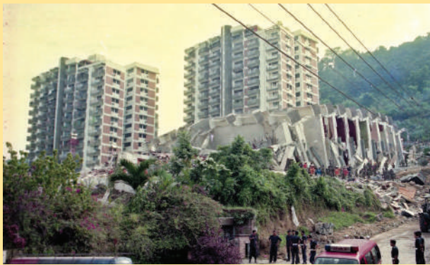
Ampang, Highland Tower Collapse, 1993
