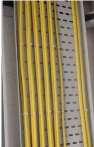
Figure 21. Vertical cable installation via open trunking
