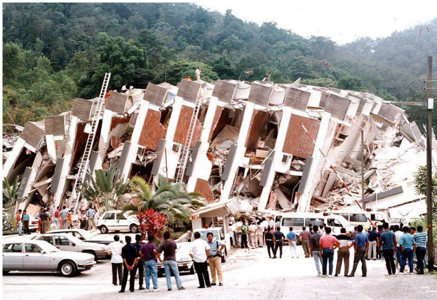
Figure 4.1 : Highland Tower incident
